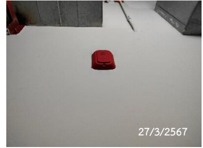
Fire Alarm Horn Strobe
