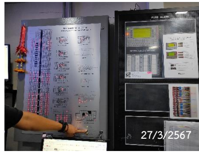
Graphic Annunciator Fire Alarm
