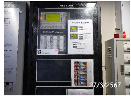
Fire Alarm Control Panel
